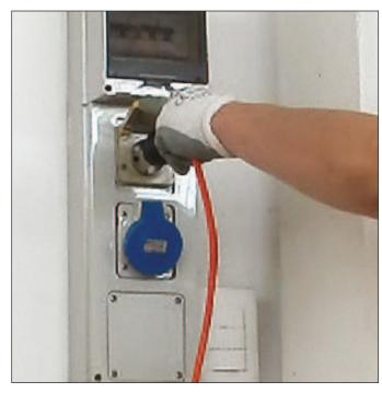
1. Check the power supply cable to see if it is damaged, faulty or disconnected from the electrical mains. (\*)
